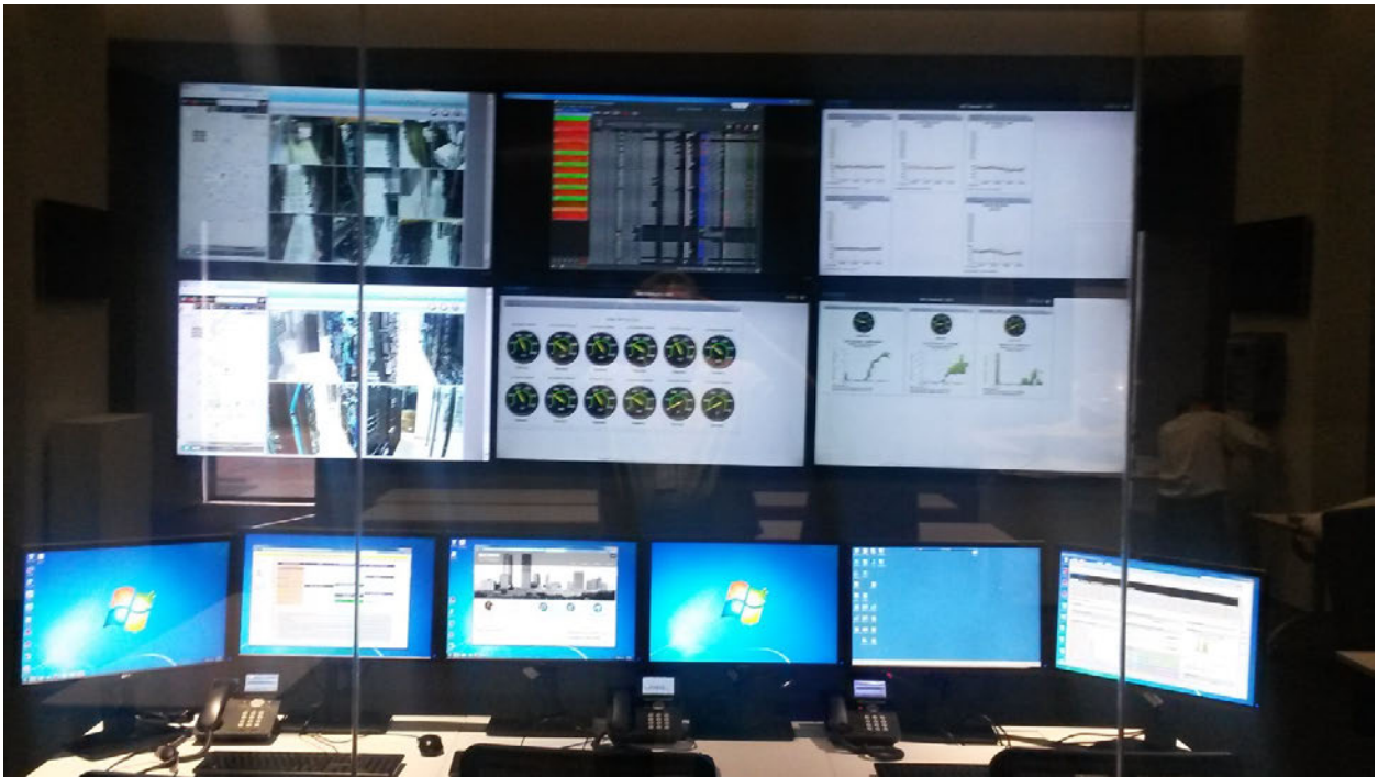
Securus Backup Network Operations Center
